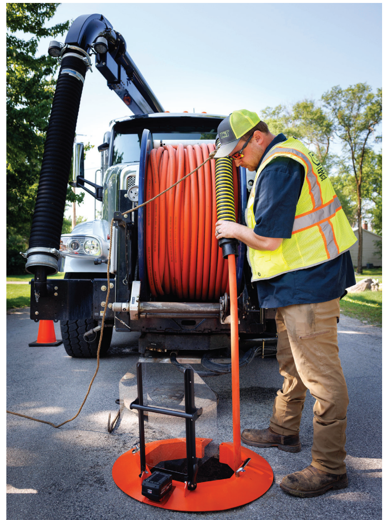
▲ CIT Sewer Solutions equipment manager Eric Johnson uses a Vactor 2100 to clean a sewer line.
